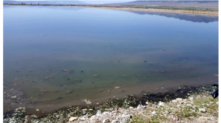
Figure 1. 0.4 MGD lagoon system after a toxic hit. The wastewater color was milky, with floating solids indicating biomass die-off.
