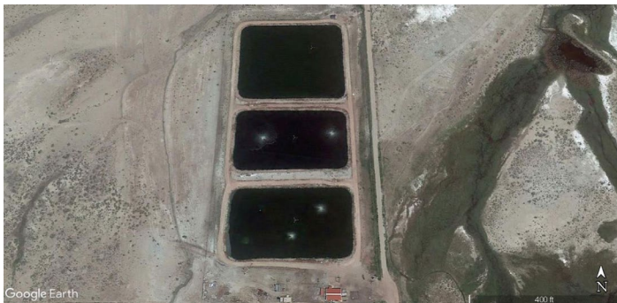
Figure 1. Google Earth image of the 0.3 MGD wastewater lagoon system.
