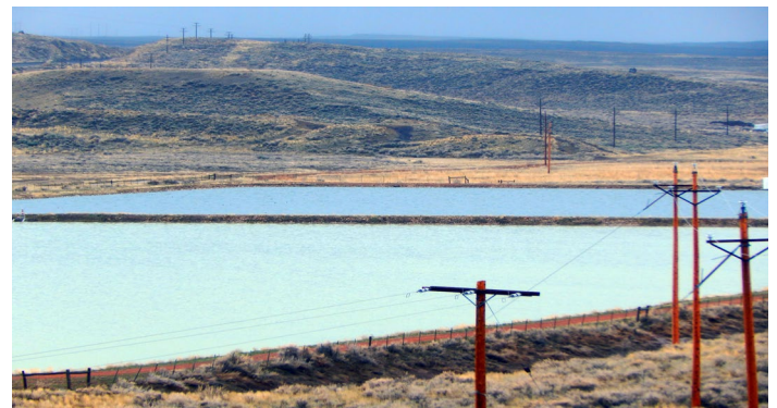
Figure 2. Two-cell facultative lagoon system serving a rural Wyoming municipality.
