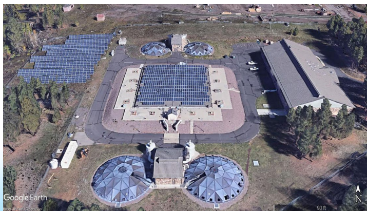
Figure 1. Google Earth image of the 2 MGD ASP experiencing washout events due to I&I.
