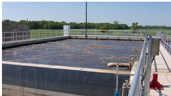
Figure 1. A sequencing batch reactor similar to the one located at the plant. A strong-smelling odor was emitted from the plant during periods of low flow in the late winter months.
