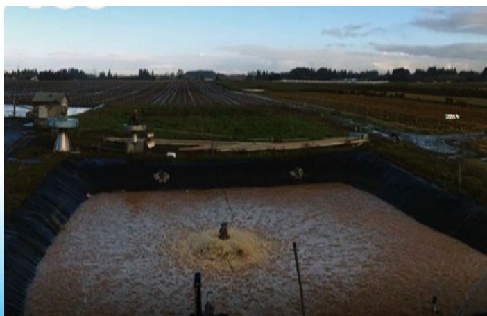
Figure 1. Case study wastewater treatment system encompassing mechanical, clarifier, and lagoon components.
