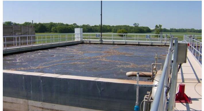
*Figure 1. A sequencing batch reactor similar to the one located at the plant. A strong-smelling odor was emitting from the plant during times of low flows in the late winter months.*
